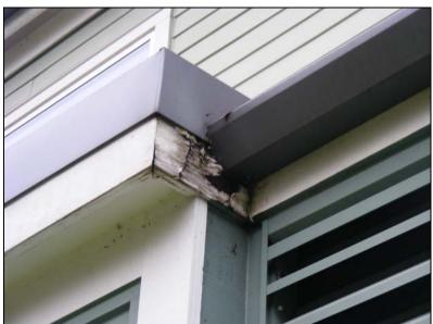
Exterior finish – wood trim is failing.
